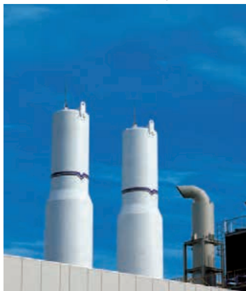
Oxygen supplied from liquid oxygen tanks is used in the oxy-fuel firing furnaces
