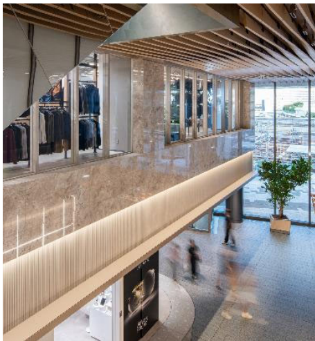
Heat-resistant laminated glass windows convey the atmosphere of the lower floors while ensuring clear visibility and safety.
